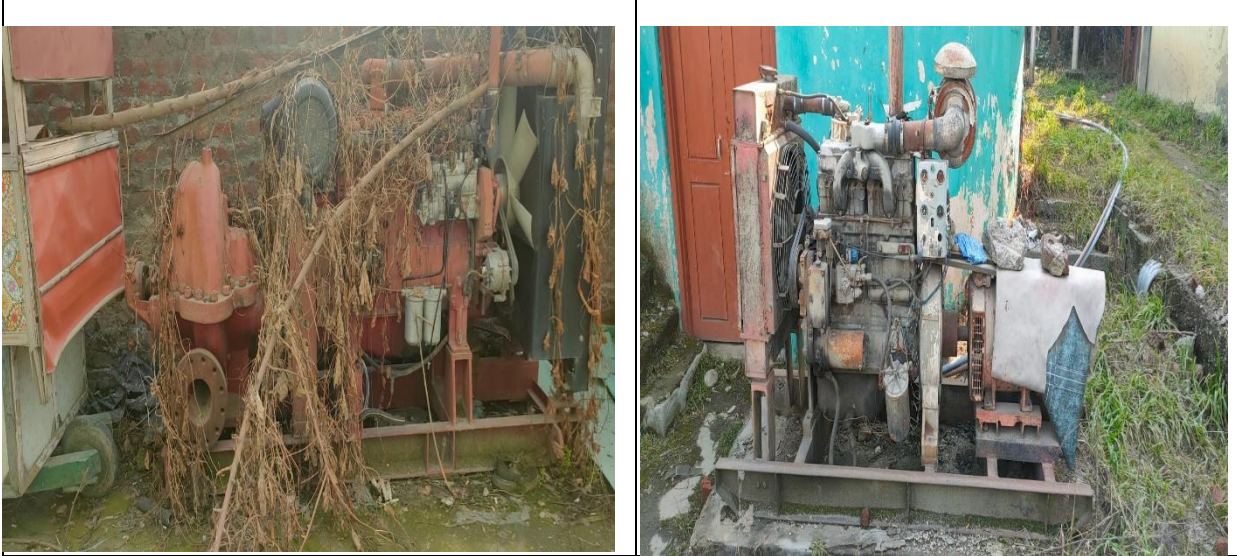
THEN: Inefficient Diesel Generators operating at temporary Pumping Stations
