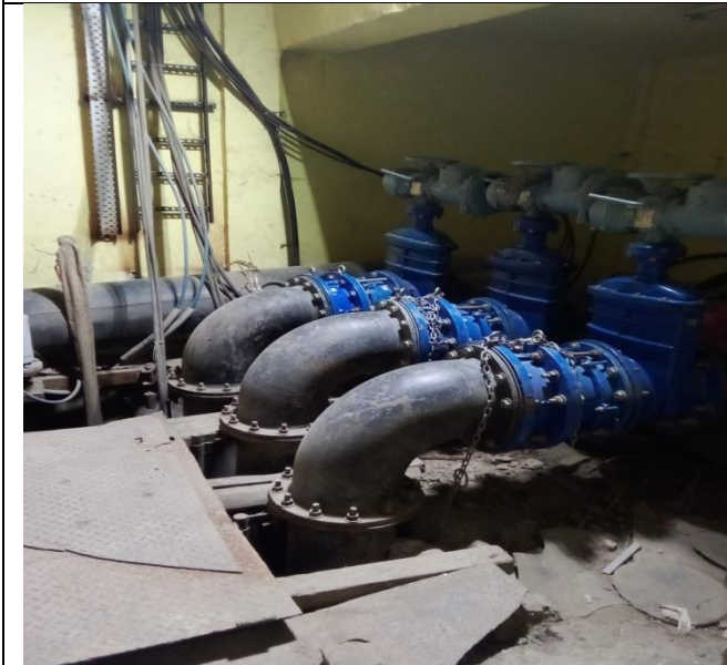
Actuators & Valves installed at Sump well
