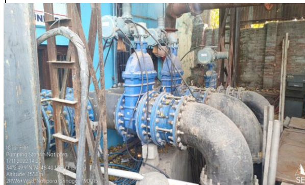
Now: Pipes upgraded with submersible pumps
