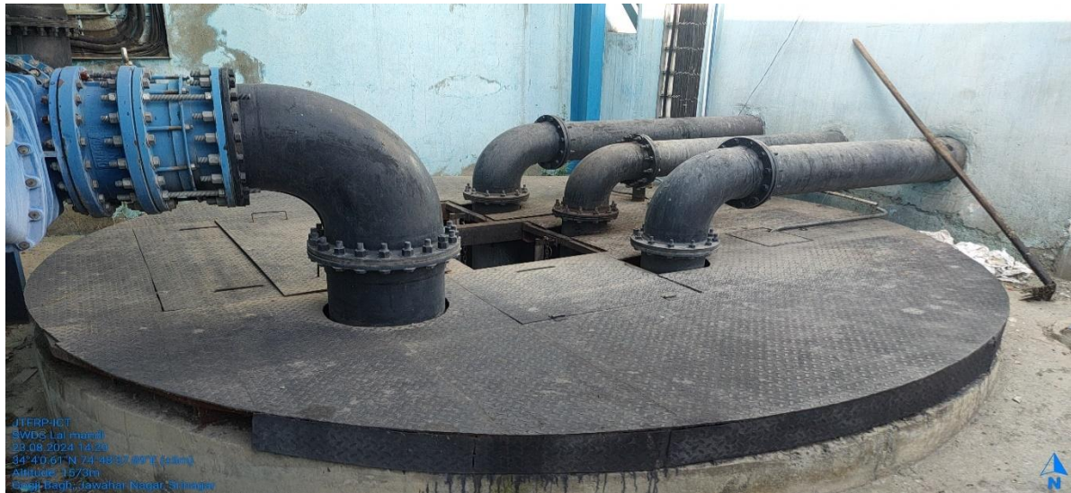
A view of Securely covered sump with chequered plate and neatly painted pipes ensuring drainage efficiency and corrosion protection at Dewatering Stations
