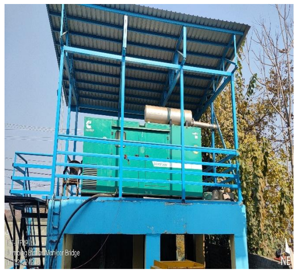
THEN: Inefficient Diesel Generators operating at temporary Pumping Stations
