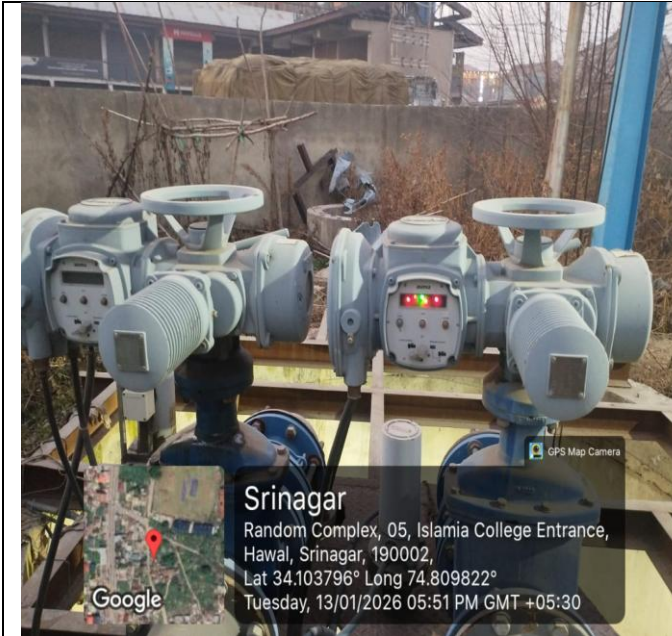
Actuators installed at Sump well
