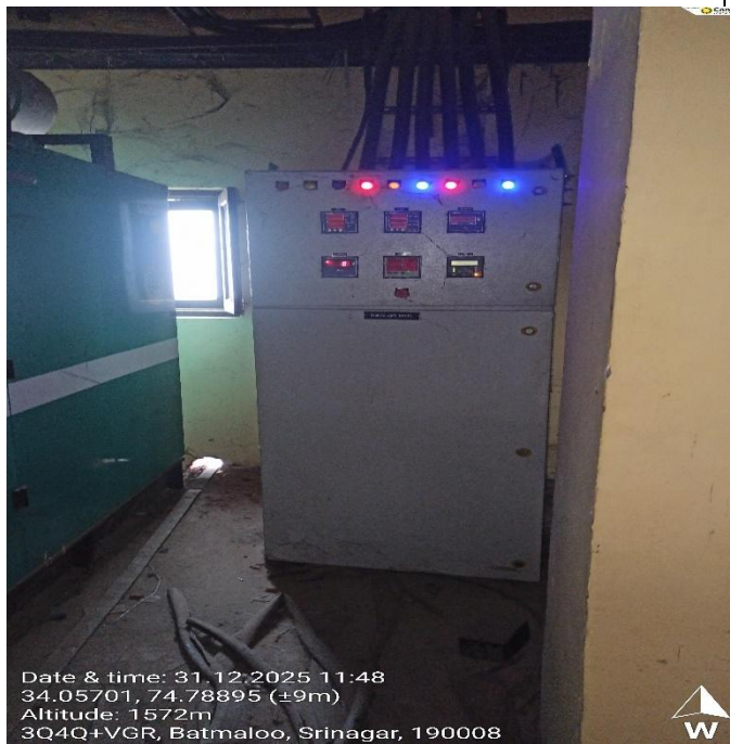
Installation of AMF Panel inside control room located in first floor of pumping station which is above HFL 2014
