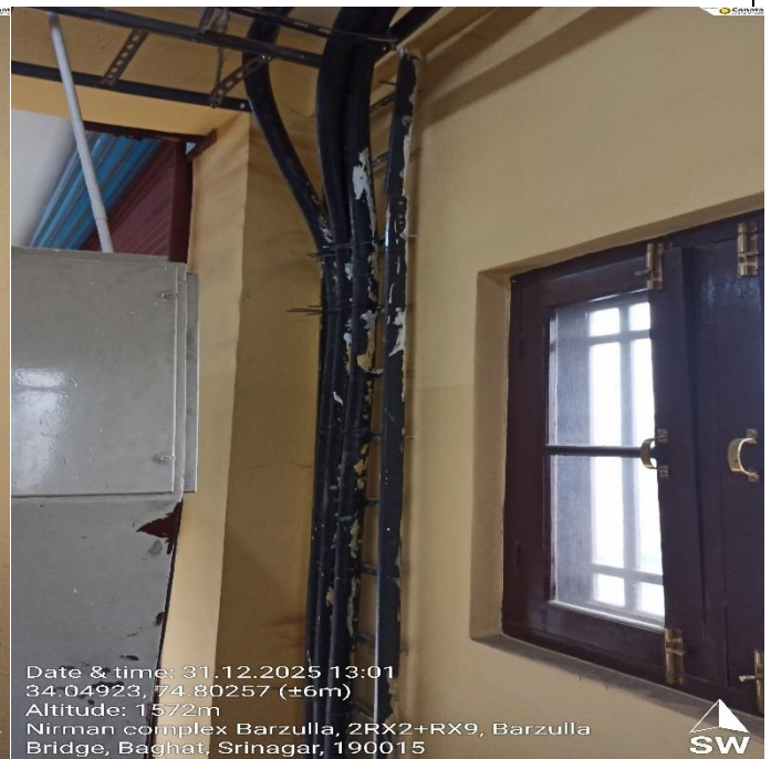
Cable Management Through cable ladders and trays inside the control room
