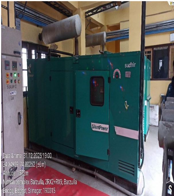
Installation of DG Set inside control room located in first floor of pumping station which is above HFL 2014
