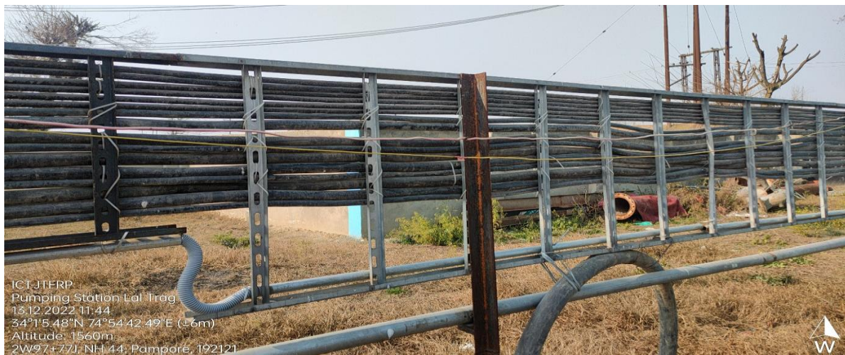
Electric cables neatly routed on ladder trays for safe and organized distribution at Dewatering stations
