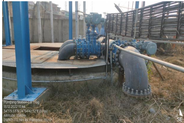
NOW: Energy efficient submersible pumps installed
