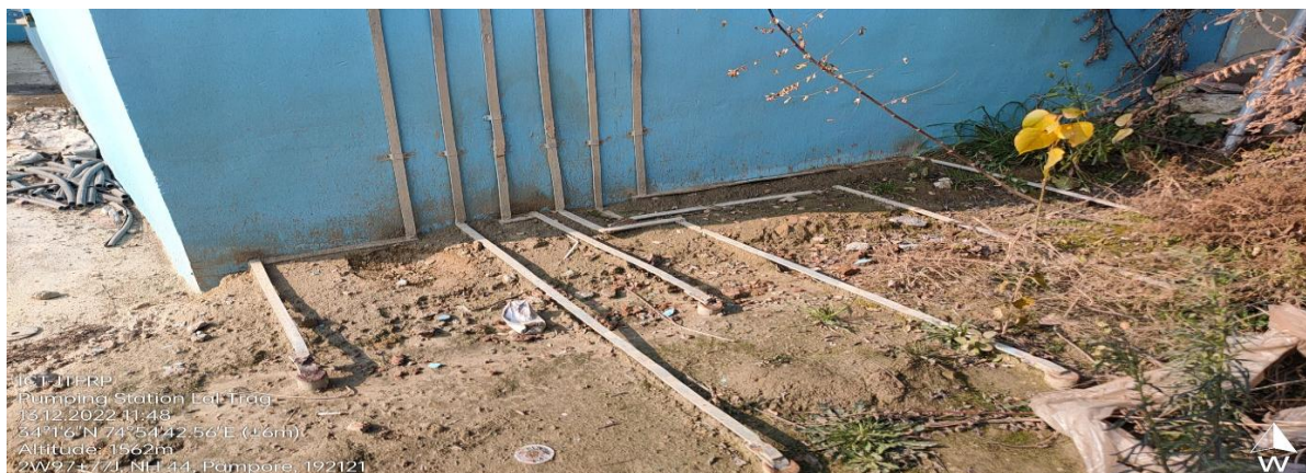
Properly installed earthing strips and rods ensuring low-resistance grounding for electrical safety at Dewatering stations.
