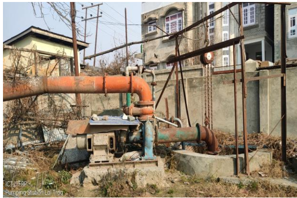
THEN: Old inefficient pumps installed at Lal trag Dewatering station
