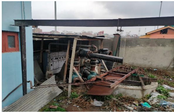
Then: Condition of Radpora Dewatering station. Sumps uncovered
