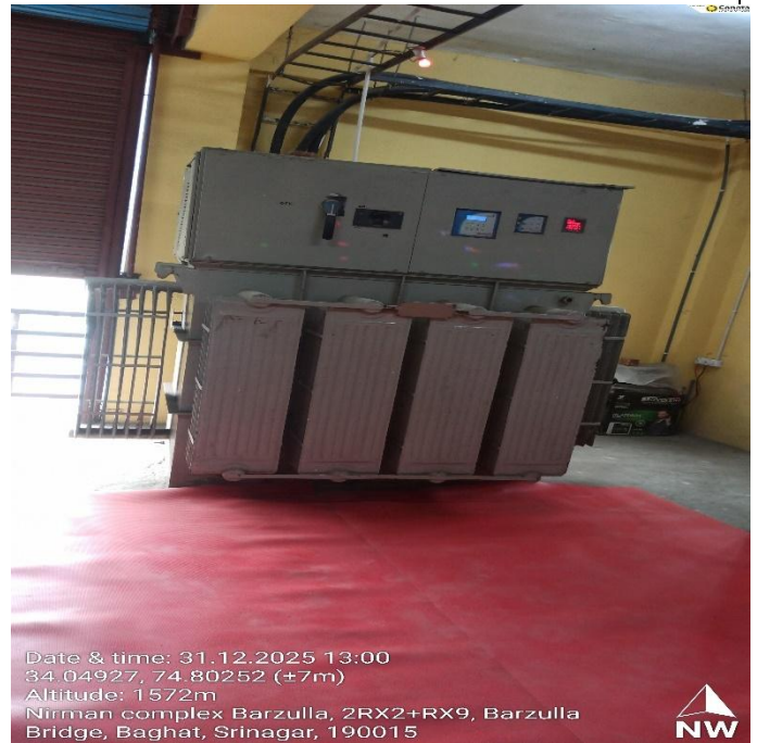
Installation of Servo Stabilizer inside control room located in first floor of pumping station which is above HFL 2014
