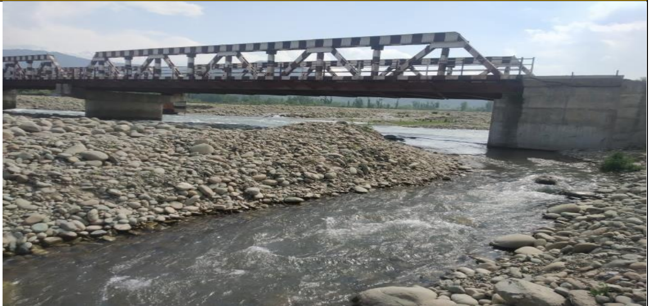
A surviving span of the Chambgund bridge over the Veshaw Nallah, which remained intact and structurally resilient during the devastating September 2014 floods, while the adjoining temporary causeway was completely washed away.
