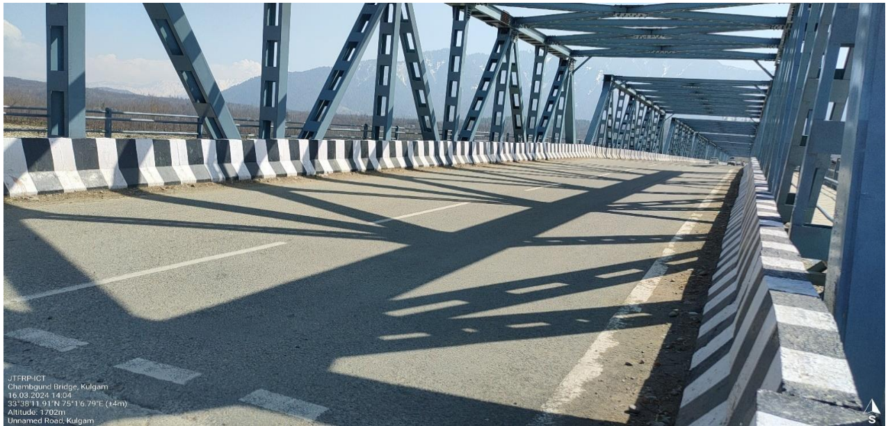
A view of the Chambgund Bridge superstructure showing the composite steel truss girder system, longitudinal girders, Bituminous top, and safety parapets
