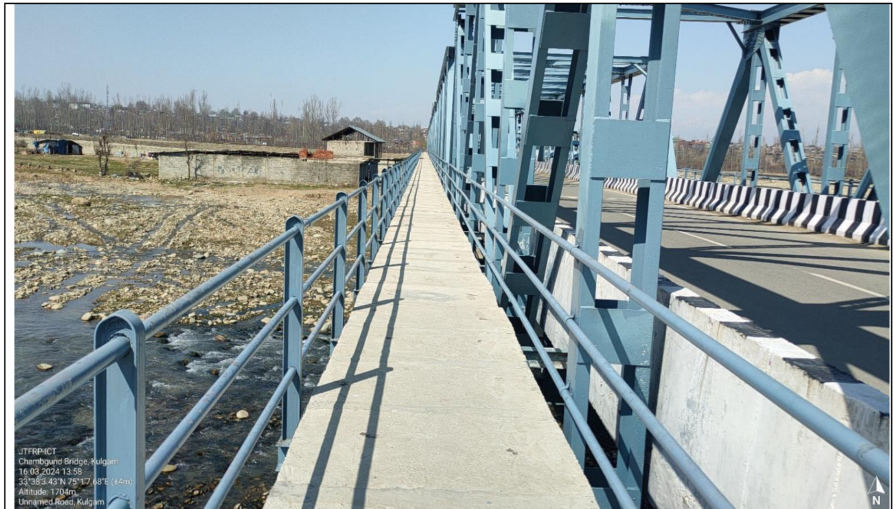
A view of 1.50m wide footpath on both sides of the Chambgund bridge, Kulgam
