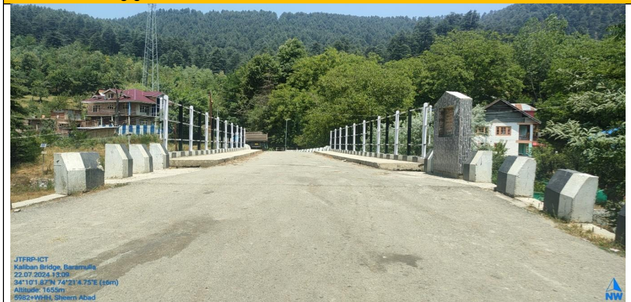
A view of the Kaliban Bridge superstructure showing the carriage way with Bituminous to beam with railing guard.
