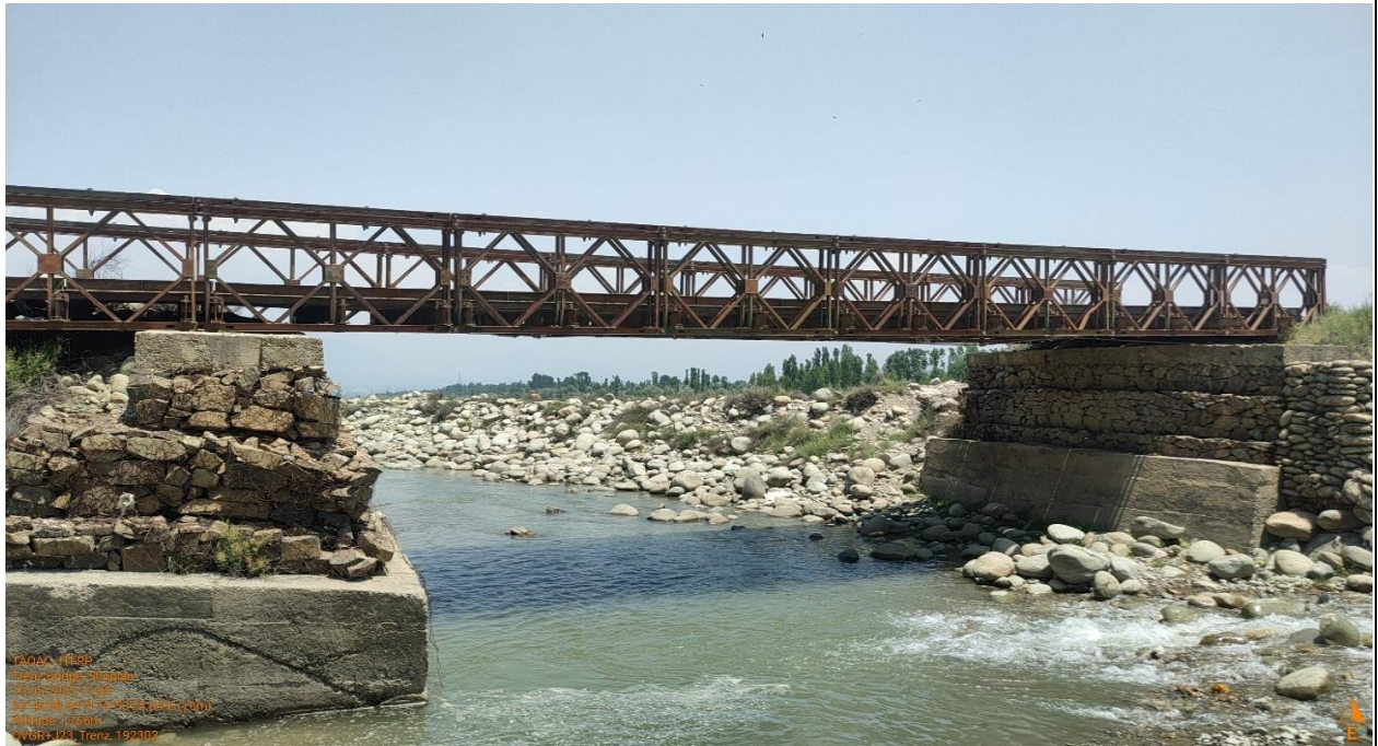
A view of two short span bailey bridges that were existing before the construction of the new Trenz Bridge, Shopian
