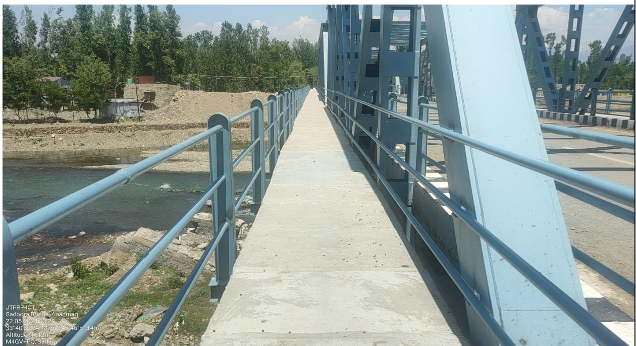
A view of 1.50m wide footpath on both sides of the Sadoora bridge at Anantnag.
