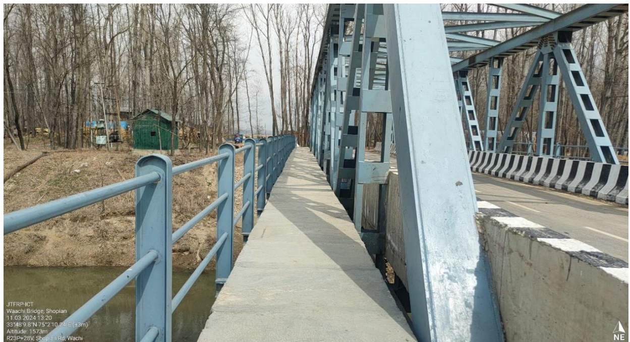
A view of the 1.50 m wide footpaths constructed on both sides of the Wachi Bridge.
