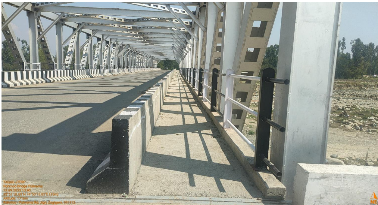
A view of 1.50m wide footpath on both sides of the Rohmoo bridge.
