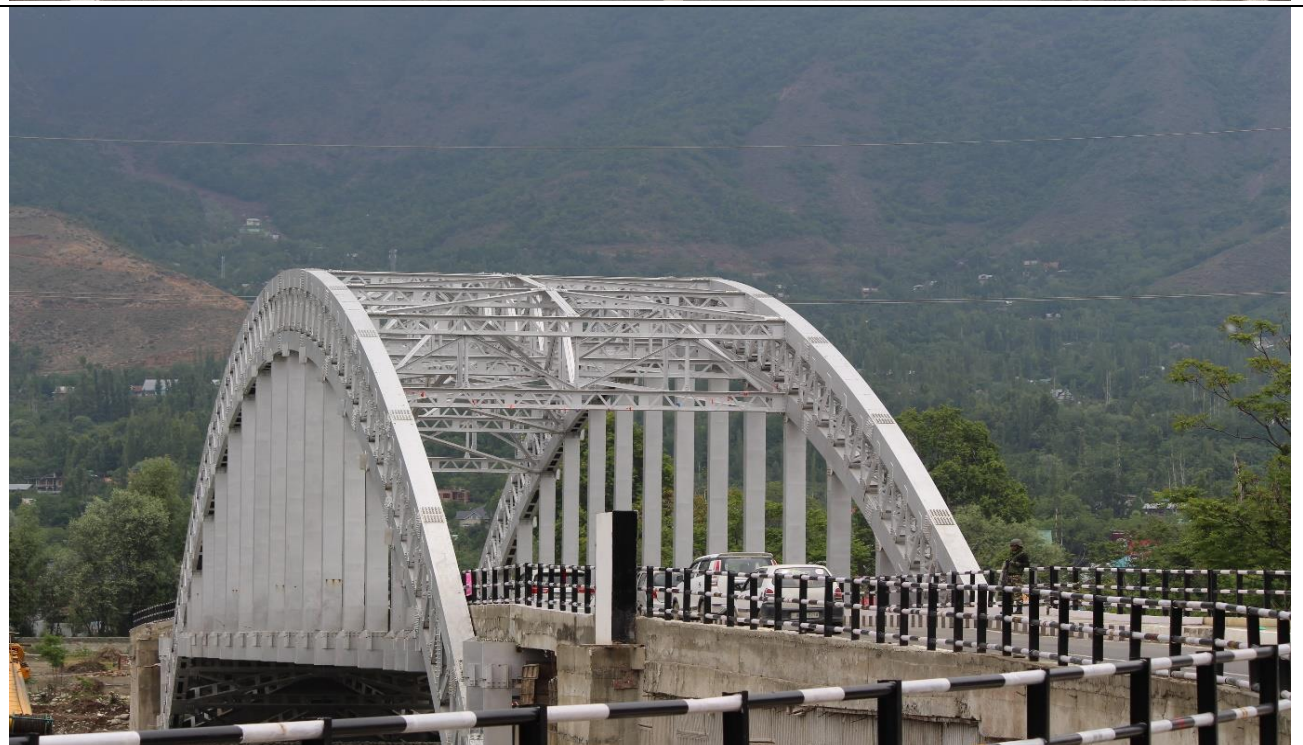
Views of the Wayil Bridge superstructure showing the composite Semi arch steel truss system, longitudinal girders, deck slab, top bracing, Bituminous top, and footpaths.
