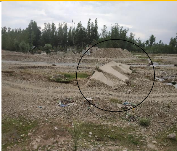
Views of remnants from the previously damaged Sadoora Bridge at Anantnag, illustrating the extensive structural deterioration and debris left by recurrent flooding events prior to the JTFRP reconstruction efforts
