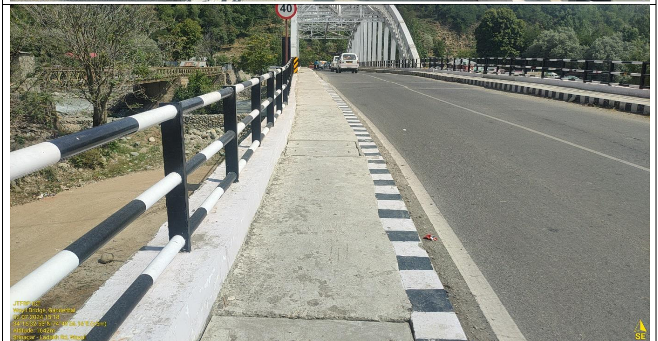
A view of 1.50m wide footpath on both sides of the Wayil bridge
