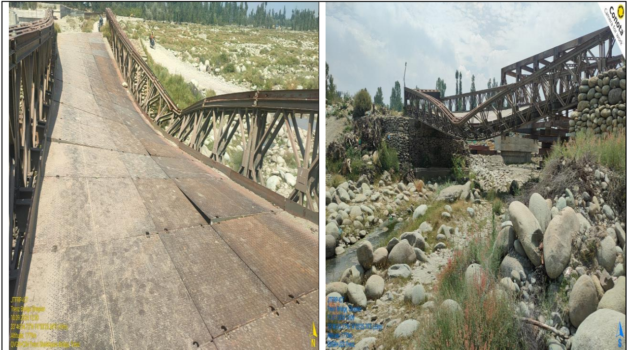
Photograph showing the damaged Bailey bridge at Trenz, affected by flash floods prior to the construction of the new resilient bridge.
