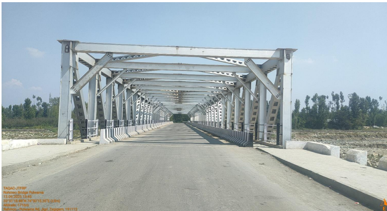
A view of the Rohmoo Bridge superstructure showing the composite steel truss girder system, longitudinal girders, Bituminous top, and safety parapets
