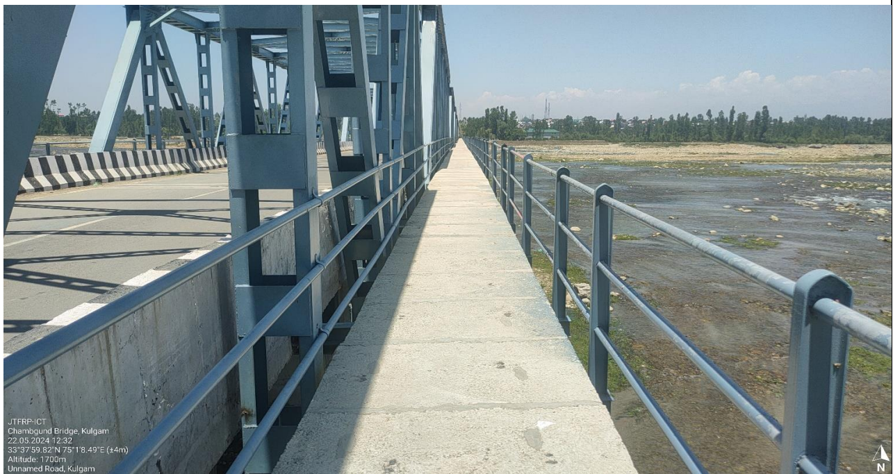
A view of the Chambgund Bridge superstructure showing the composite steel truss girder system, longitudinal girders, Bituminous top, and safety parapets
