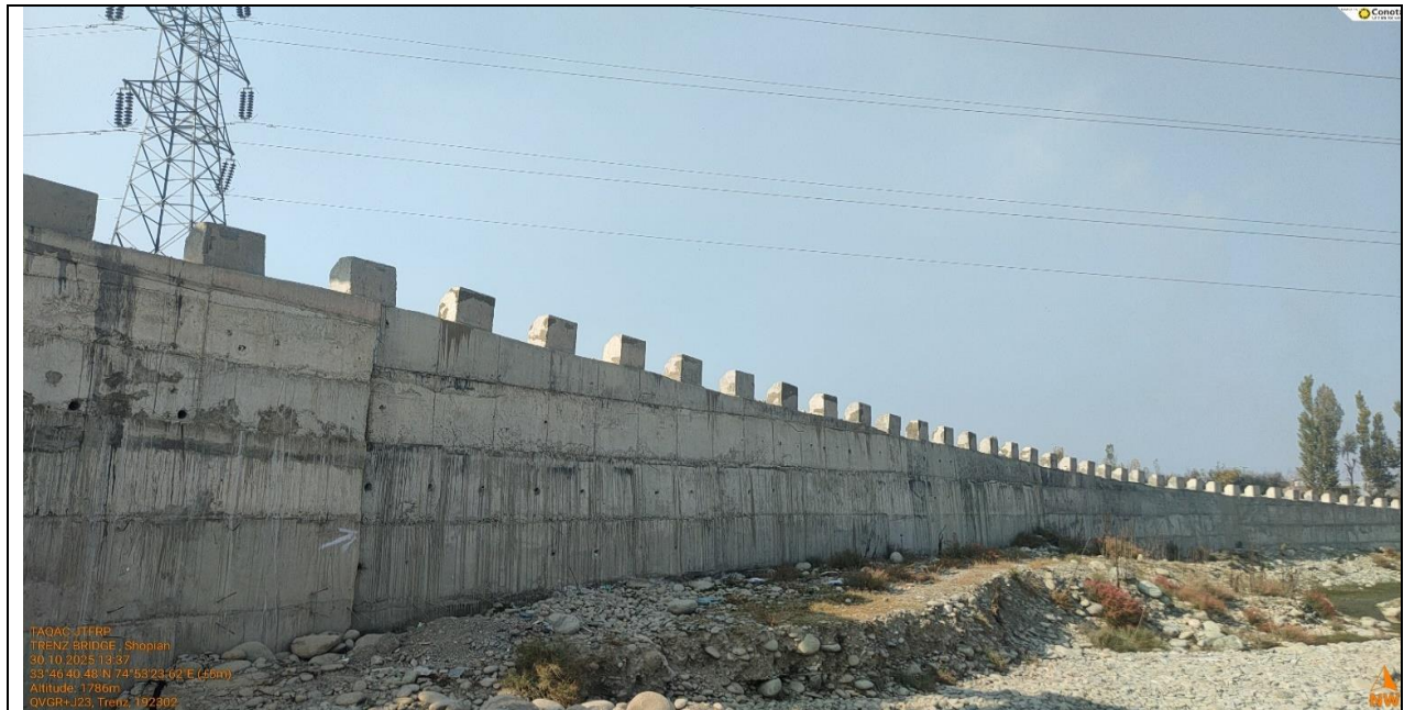
A view of Approach retaining wall with parapets
