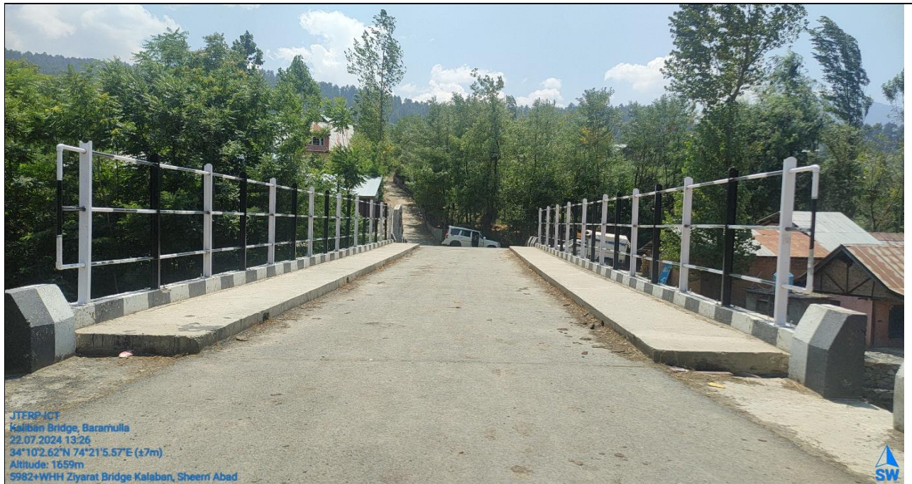
A view of the Kaliban Bridge superstructure showing the carriage way with Bituminous to beam with railing guard.
