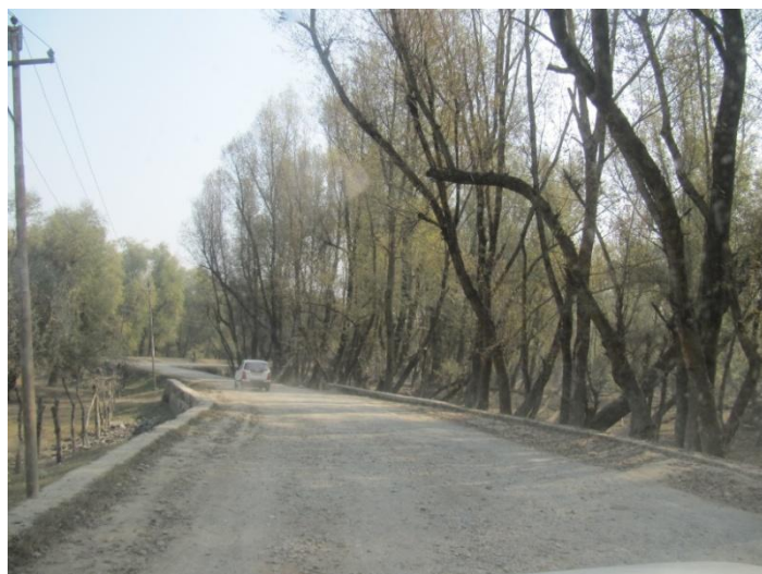
Existing conditions of Sub-project road
