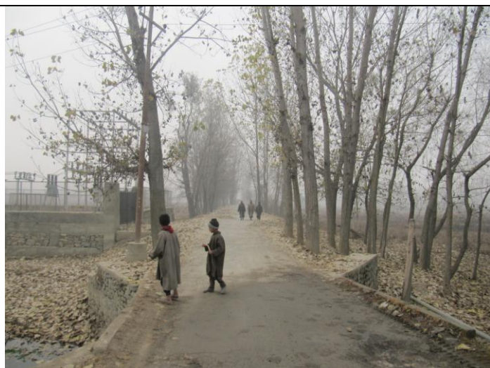
Culvert in road alignment
