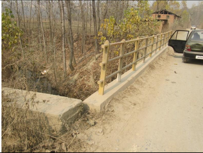
Culvert on irrigation canal crossing subproject road
