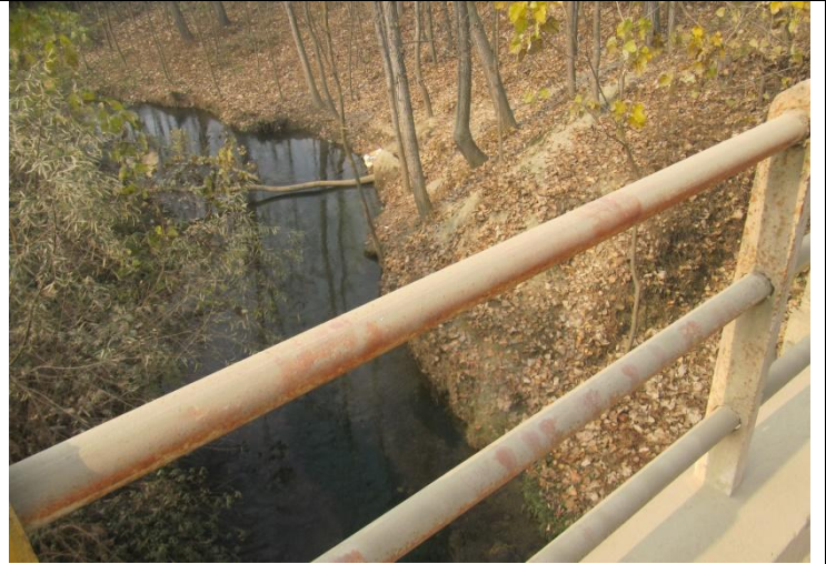
Culvert on irrigation canal crossing subproject road
