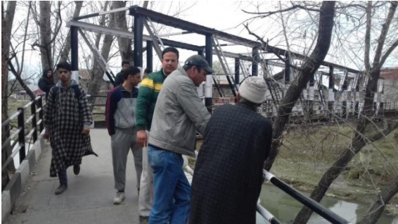
Chhanpora Sluice Station
