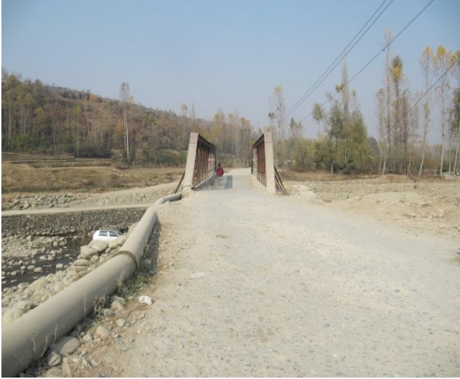
Existing Bridge on NingliNallah & PHED pipeline
