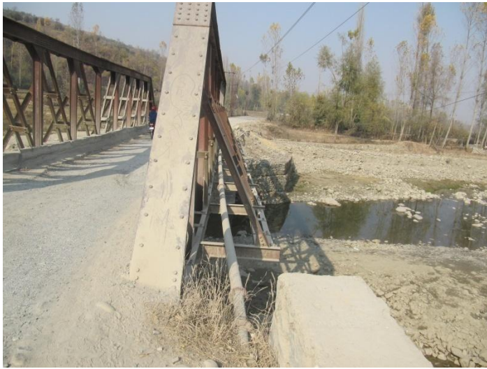
Water supply pipeline on existing bridge
