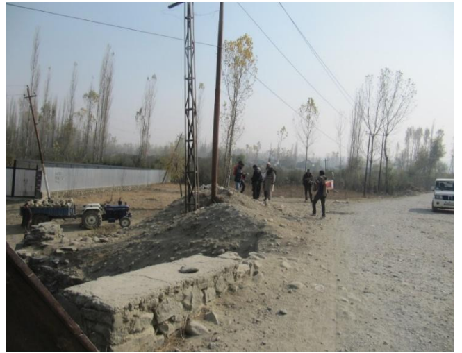
Approach and utilities.
