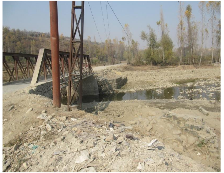
Electricity poles coming in alignment of new bridge
