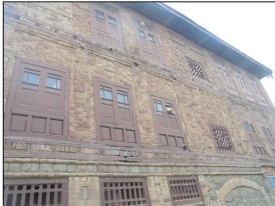
**Unreinforced brick masonry in cement mortar with reinforced concrete floor/ roof slab**
