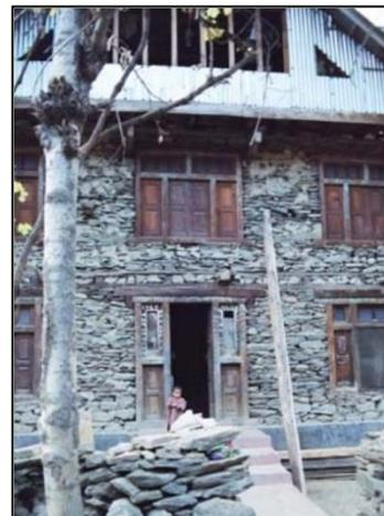
**Massive stone masonry in (lime/cement mortar).**
