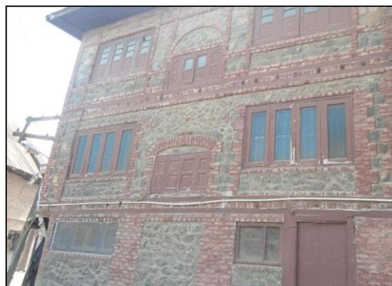
***Dressed stone (regular shape) masonry in (lime/cement mortar).***
