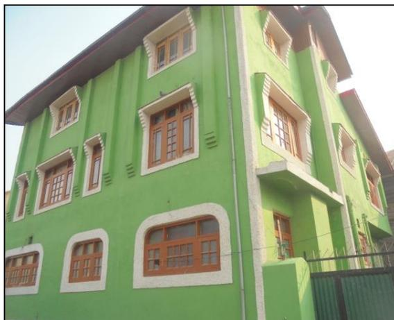
***Confined bricks/ block masonry with concrete posts/ tie columns & beams***
