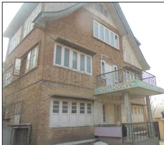
**Unreinforced brick masonry in mud mortar with vertical posts/ columns**
