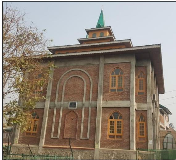
***Unreinforced lime /mud (various floor/roof) with concrete floor/slabs***
