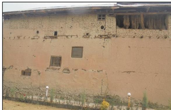
***Unreinforced brick masonry in mud/lime mortar.***
