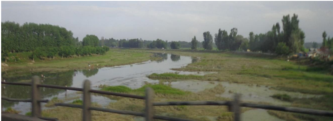
Photograph of Flood Spill Channel Reach –Near Channel Outlet to the Jhelum River – View upstream
