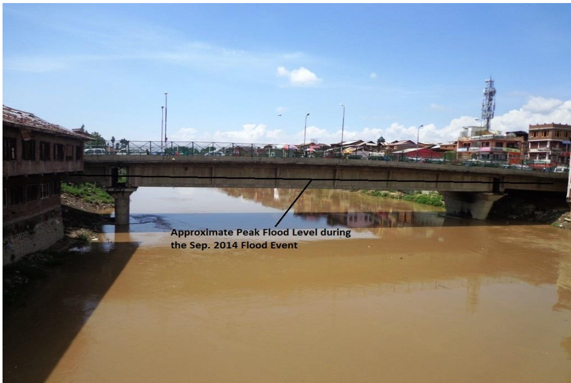
Photograph of Badapora Bridge with Restricted Bridge Deck (Soffit) Height and Width
