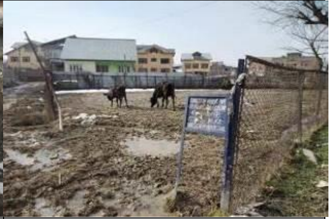
Figure 4-5: Intermediate Pumping Station at Bonpora.
