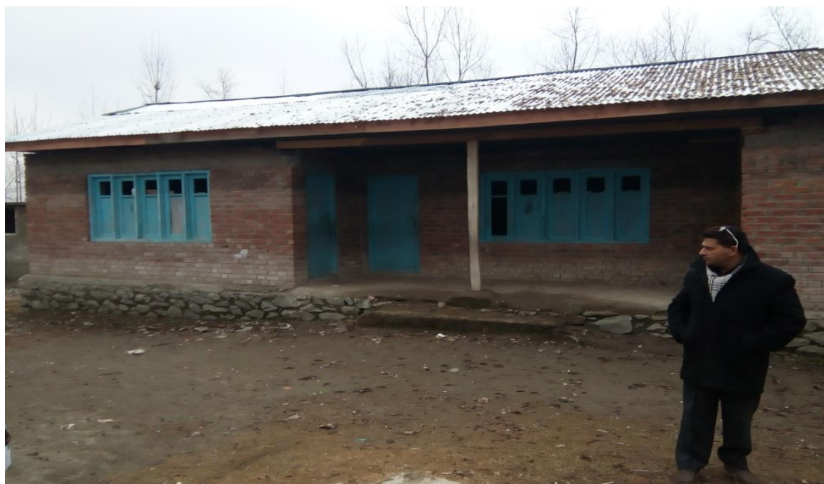
Existing School Building
