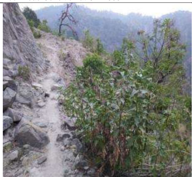
Foot track Road at Ch.3.500 Km
