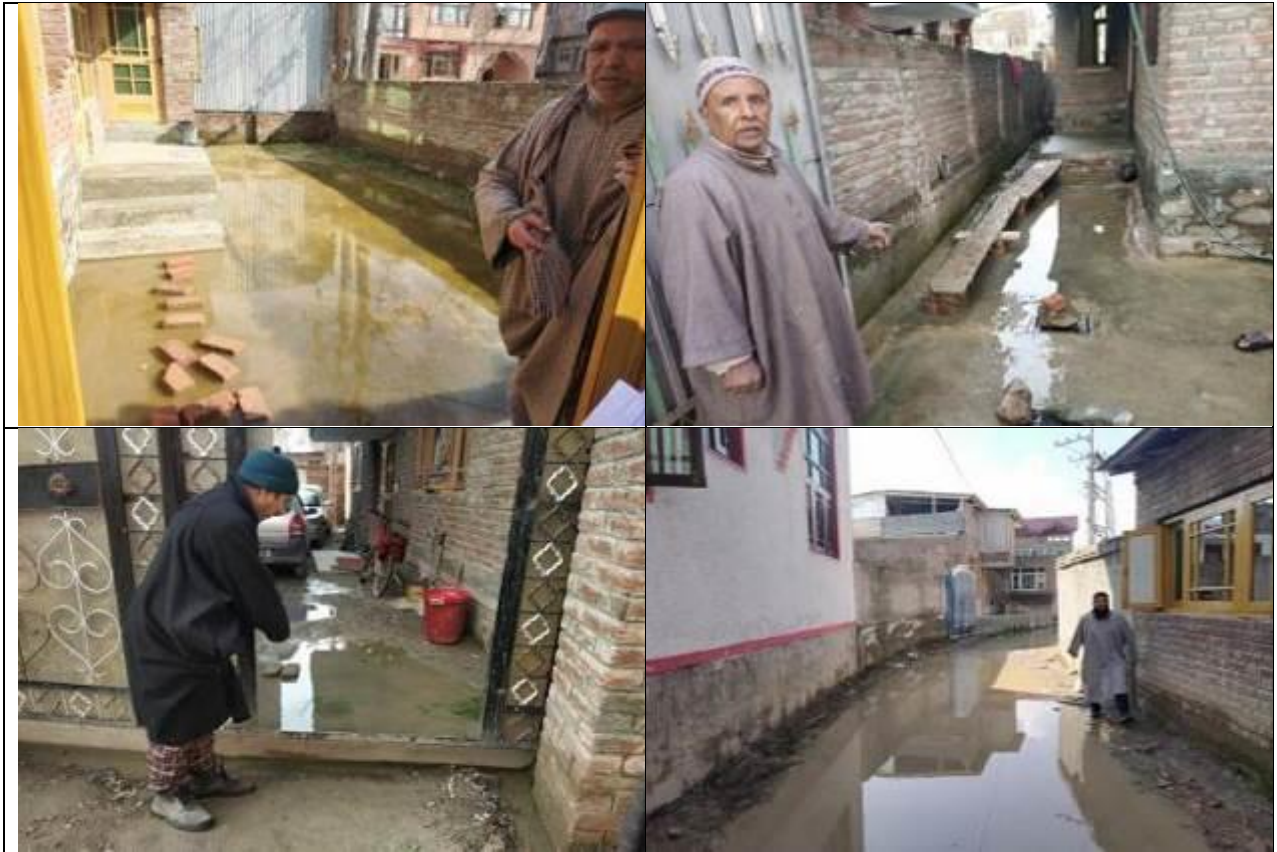
Figure 4-2: Submergence/ waterlogging of houses, lawns, roads is common scene during site visit.
