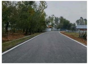
includes upgradation of road from single lane to the intermediate lane configuration in (Shadipora-Khanpeth-Sumbal ) & (Hajin –Ajas) and strengthening of existing Hamray – Sultanpora –Nowgam road with the laying of GSB (granular sub-base), WBM (wet bituminous macadam) , BM (bituminous macadam) and construction of drainage structures and protection works wherever required.
