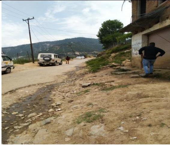
Village Thalella at Ch 3.000 Km
