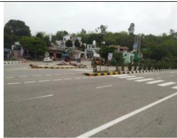
Project road starts at Sidhra (view from NH44)
