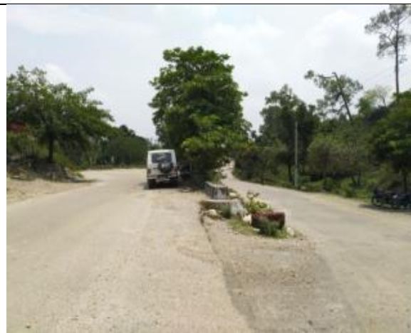
Road Side Temple at Ch10.300 RHL
