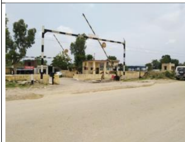
The railway crossing (at Ch 3.150 Km Bajalta)
