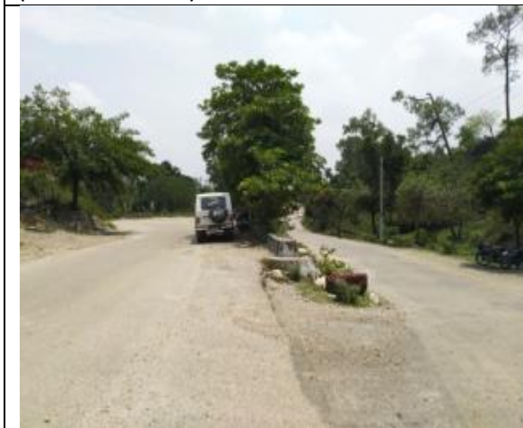
Crossing of Tutian Di Khui road at Ch 6.400 Km
