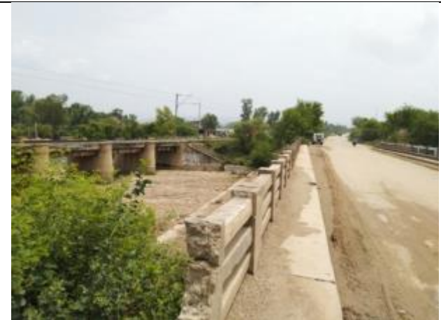
A bridge and a railway track (at Ch 2.950 Km)
