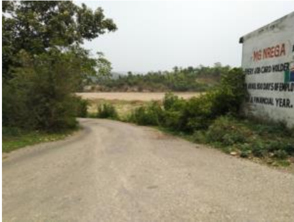
Bushes close to the road At Ch 0.700 Km
