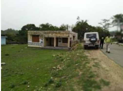
Panchayat House at Ch 2.600 LHS
