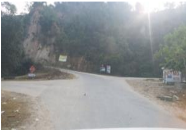
Four legged junction at Ch 1.950 Km
