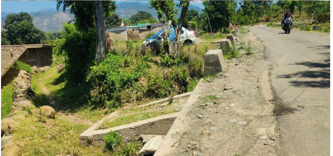
Access provided at two locations/ Pathway (300 years old restored)
