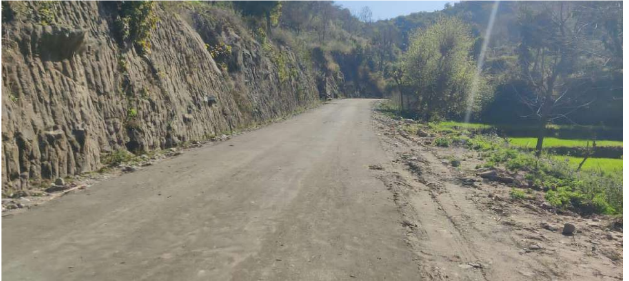
Excavated Material removed from the site
