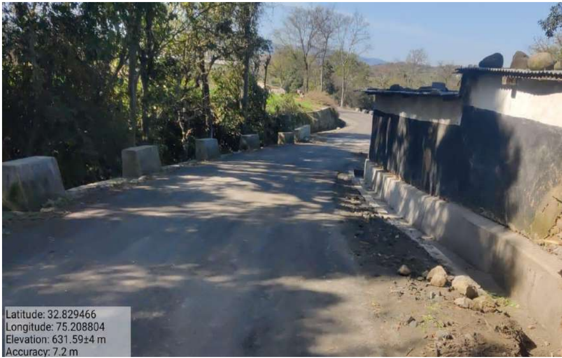
Drain constructed behind the house of one Mr. Kulwant Singh
