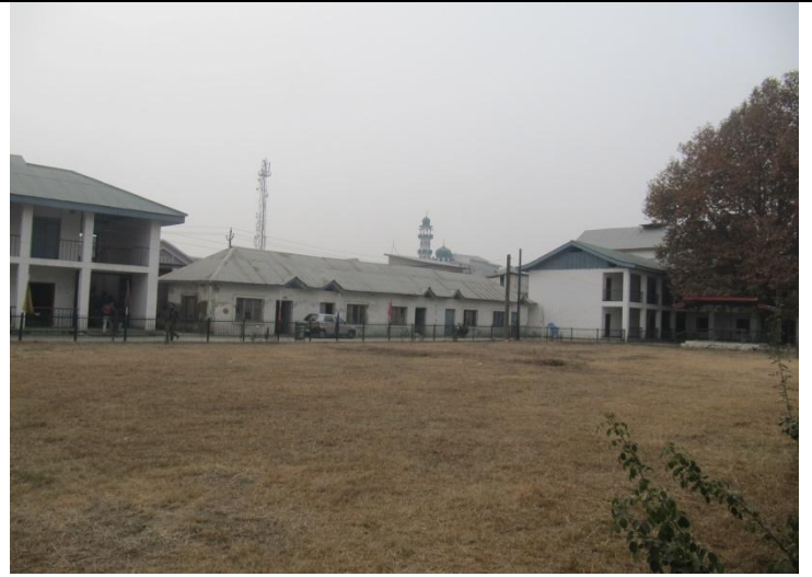
Existing damaged building in school premises
