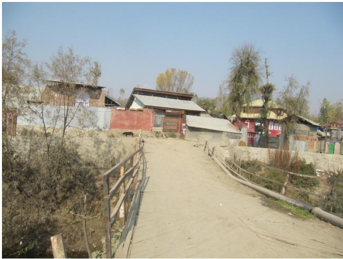
Existing Bridge and water supply pipelines
