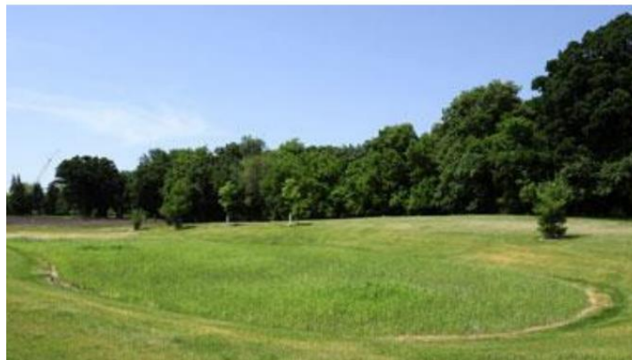
Figure 7.7: Basin for flood retention Source: EEA, 2017
