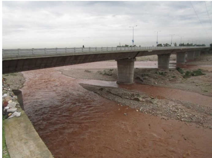
Photo 6.9: 4 th Tawi Bridge.
