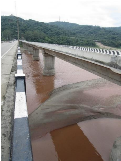
Photo 6.8: 3 rd Tawi Bridge (Sidra) near Nagrota.
