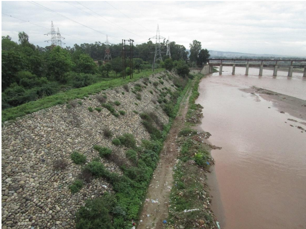
Photo 6.1: Embankment downstream of the gated section in the Waddi Tawi.
