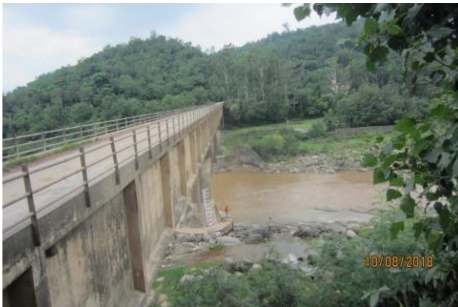
Photo 3.2: Hydrological station on Tawi River at Udhampur
