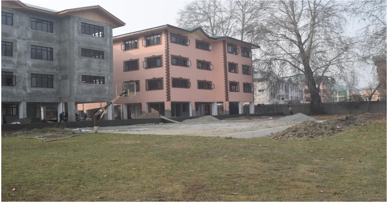
Plate.5 under construction block
