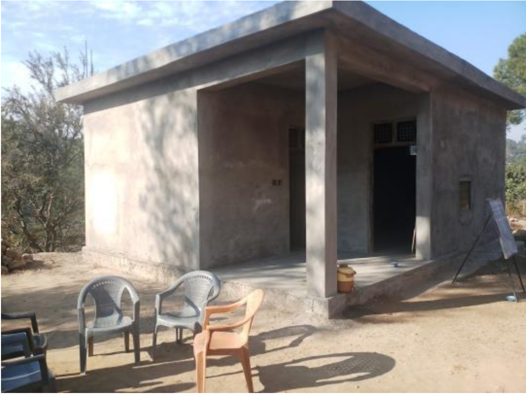
New school block under construction near proposed location
