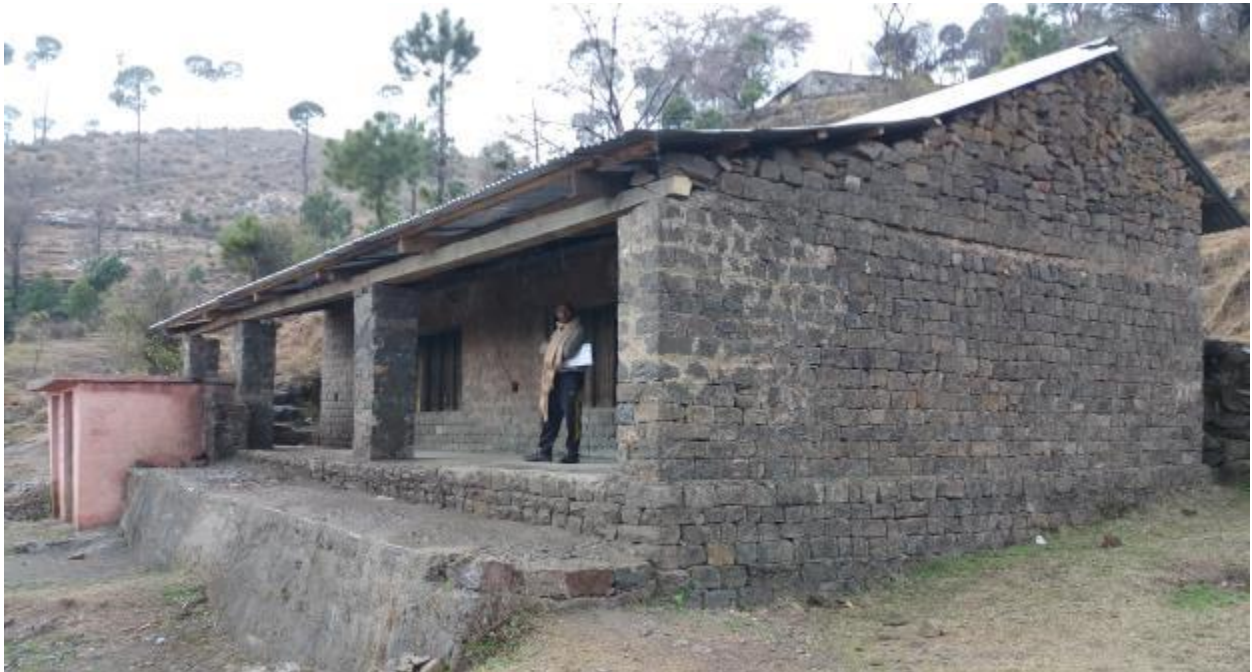
SCHOOL COMPLEX AFTER REPAIRING
