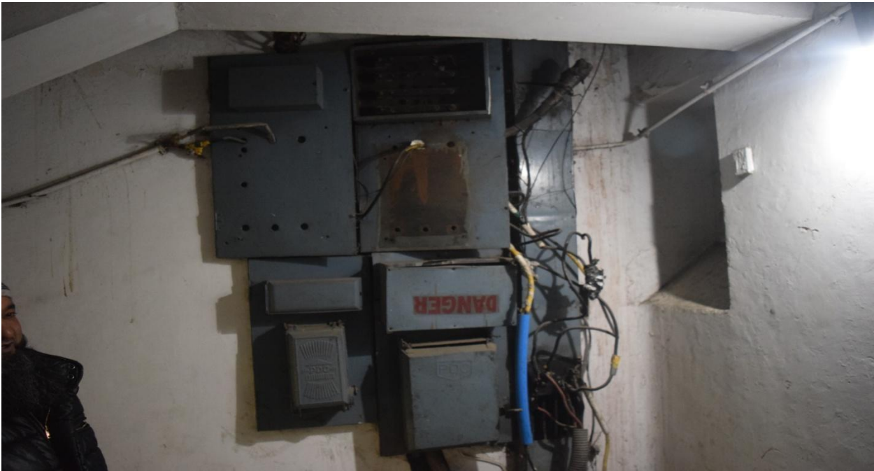
Plate.10. Electric panels posing threat to life
