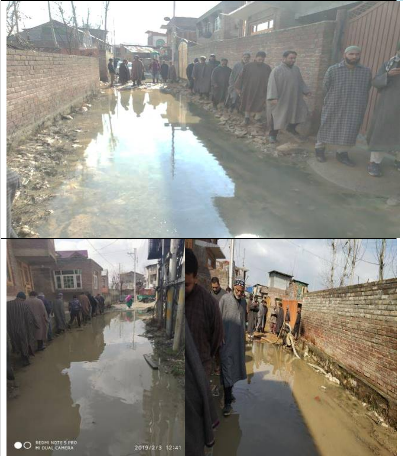
During transect walk with the community heads and the affected residents to address the sad picture of persistent submergence/ waterlogging and health hazard due to the lack of basic amenity of SWD Drainage system.
