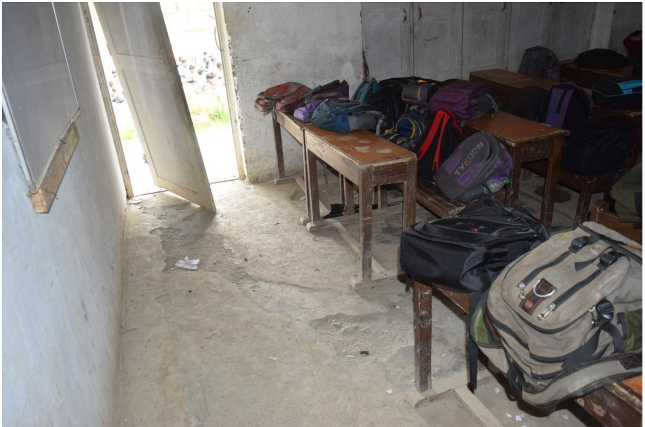
Figure 3-4: Settlement of floor as a result of floods
