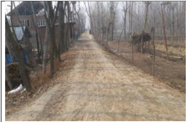
Figure 3-2: Existing Road Condition
