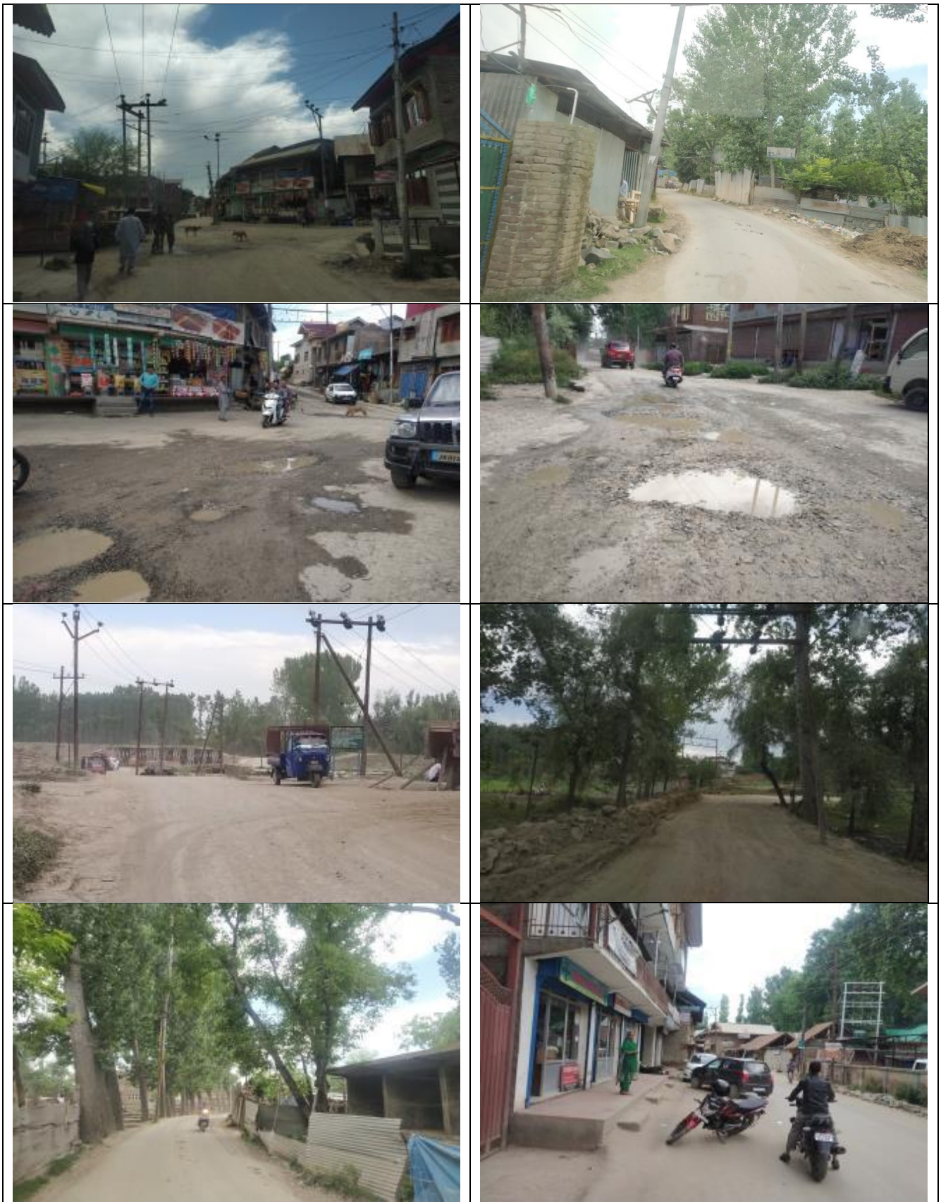
Figure 3 1: Photograph of project site
