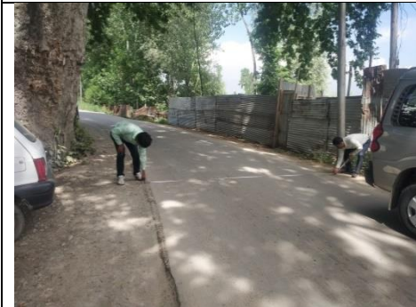
Chinar tree at RD 1+400 (RHS) is close to the road shoulder having girth class of 7.5 m. At this point ROW to be tapered towards LHS having sufficient space available to accommodate. Protective measures will be reflected in EMP/ EA report.
