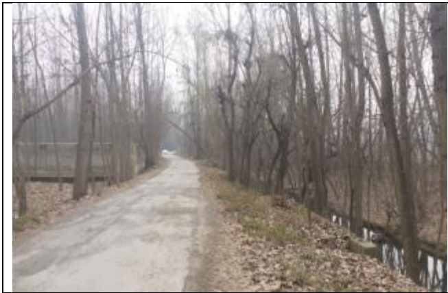
Figure 3-2: Existing Road Condition
