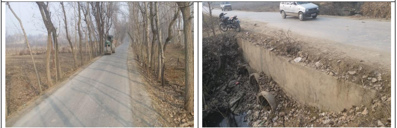
Figure 3-3: Existing Road condition
