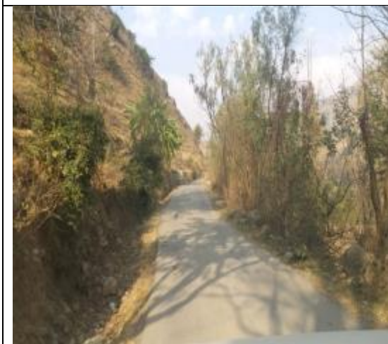
Small trees close to the Corridor at Ch 24.600 Km
