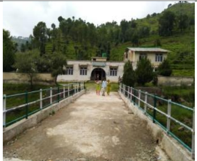
Primary Health Centre at Ch 8.100 Km LHS Gambhir Mughalan
