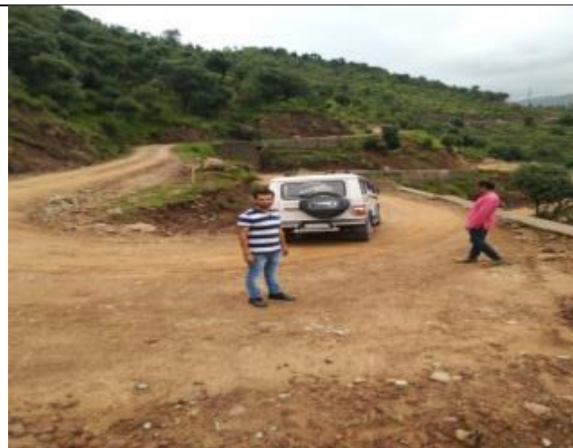
WBM road and sharp curve at Ch 16.000 Km
