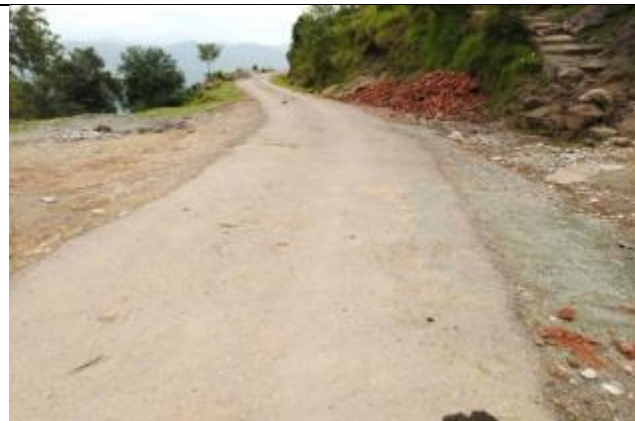
Road condition is good at Ch 11.000 Km
