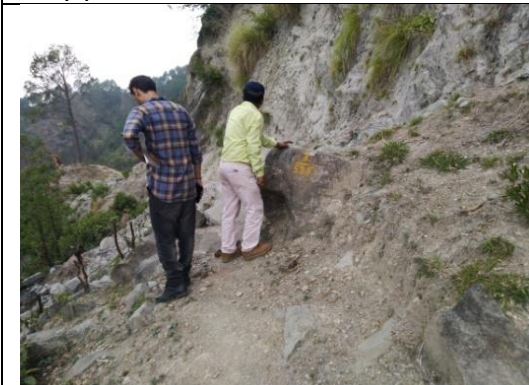
Foot track Road (Landslide prone) and landslide area at Ch 3.700 Km
