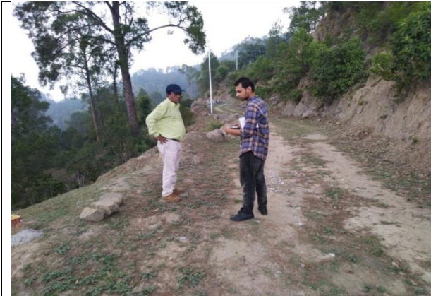
Poor Road condition at Ch 2.200 Km
