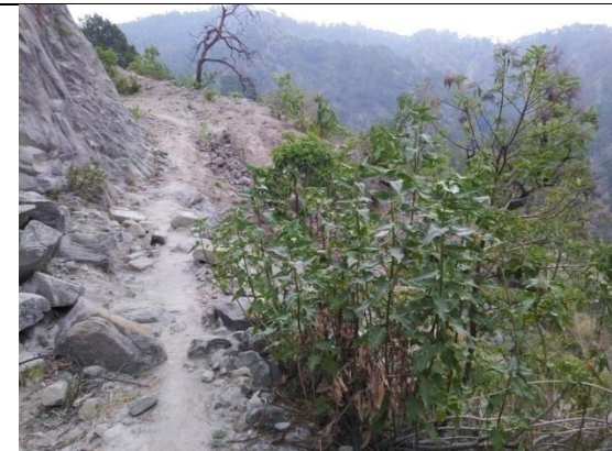
Foot track Road at Ch 3.500 Km
