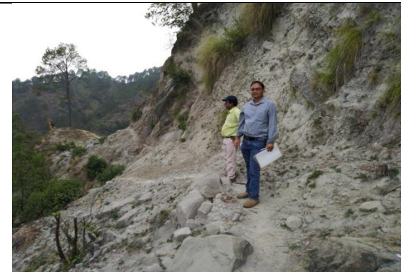
Foot track Road (Landslide prone) at Ch 3.800 Km
