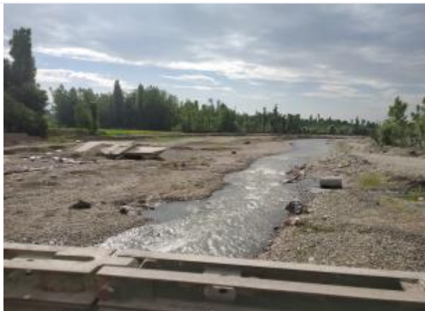
The downstream side of Brinji Nallah at Sadoora
