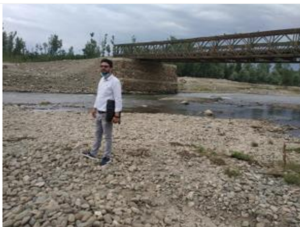
The proposed site for the bridge construction of a 3x 30-meter span bridge at Sadoora,
