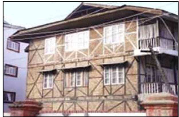
Figure 43 Dhajji Dewari House
