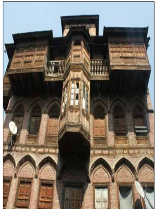
Figure 89 Traditional construction technique: Taq
