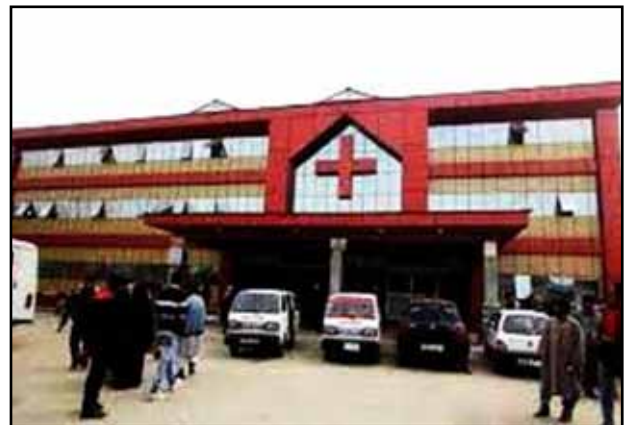
Figure 69 SMHS New Hospital clad with combustible aluminium composite panels
