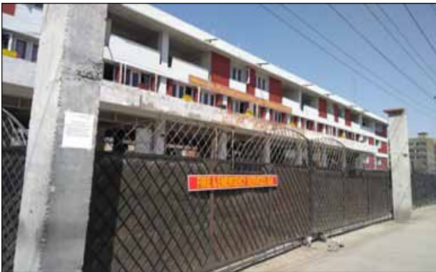
Figure 74 Fire Station at Batamallo
