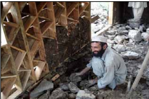
Figure 45 Construction of Dhajji Dewari House – Arup
