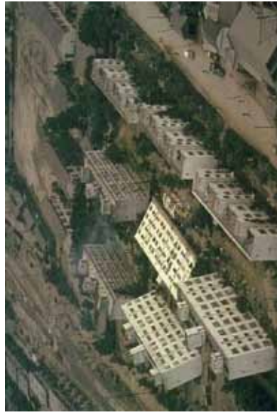
1964 Niigata Earthquake Japan
