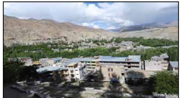
Figure 38 Urban Sprawl of Multi storey buildings in Kargil
