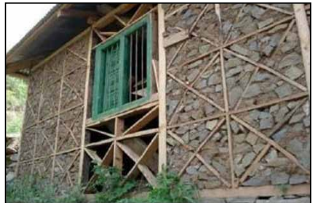
Figure 46 Completed Wall of Dhajji Dewari House – Arup
