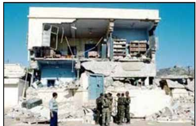
Figure 63 172 persons died in collapse of Bhuj Hospital in 2001 Bhuj earthquake
