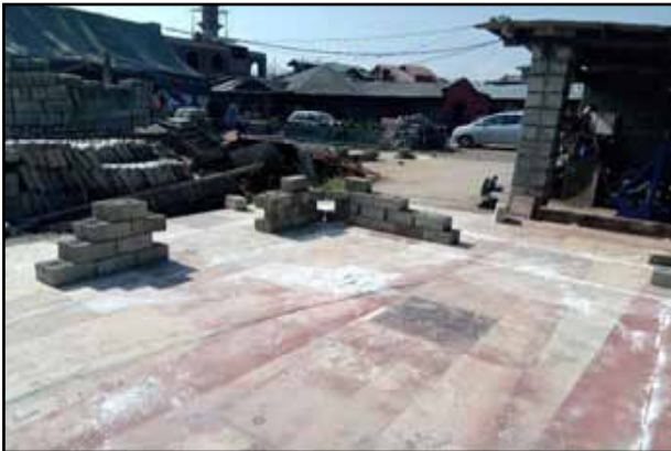
Figure 95 Practical session on Placing of confined masonry
