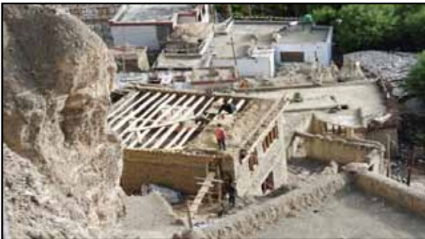
Figure 35 Traditional roof of house under construction in Leh.
