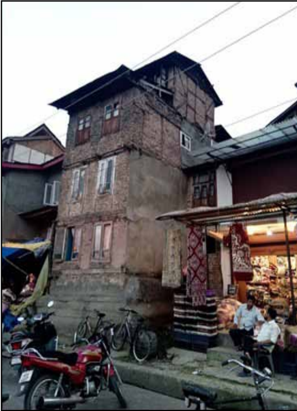
Figure 90 Traditional construction technique: Dhajji Diwari
