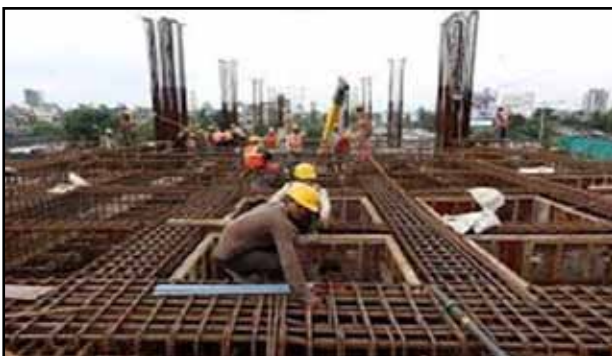
Figure 39 Reinforced Concrete Construction under quality control measures
