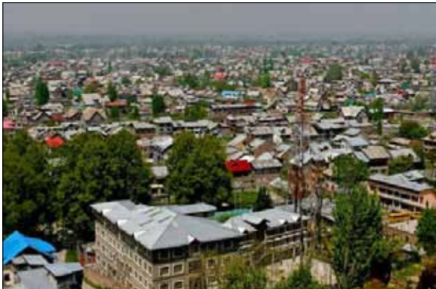
Figure 47 Development in downtown Srinagar showing closely spaced houses
