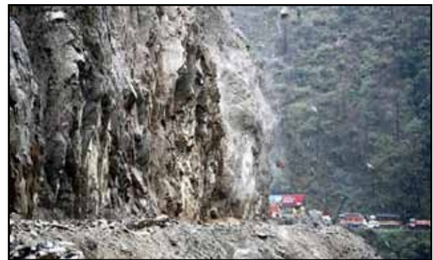
Figure 16 Landslide along Jammu-Srinagar National Highway, January 30 2019 at Ramban
