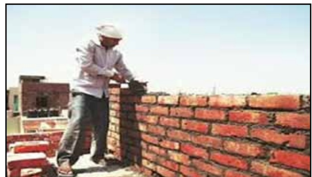
Figure 40 Load Bearing Brick wall construction
