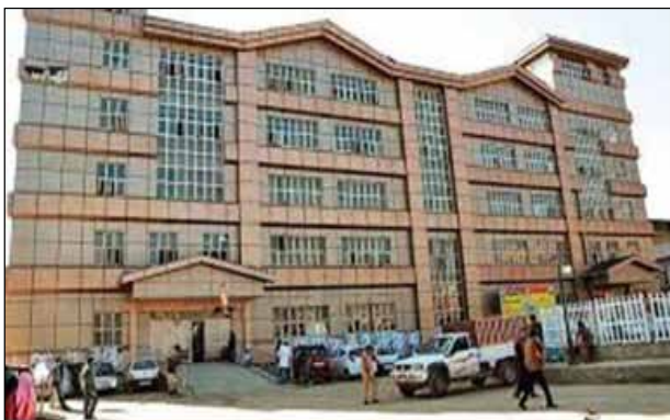
Figure 71 ACP Cladding on Lalla Ded Hospital
