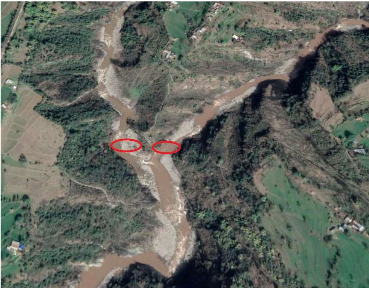
Figure 3.3: Location of bridges at the proposed site
