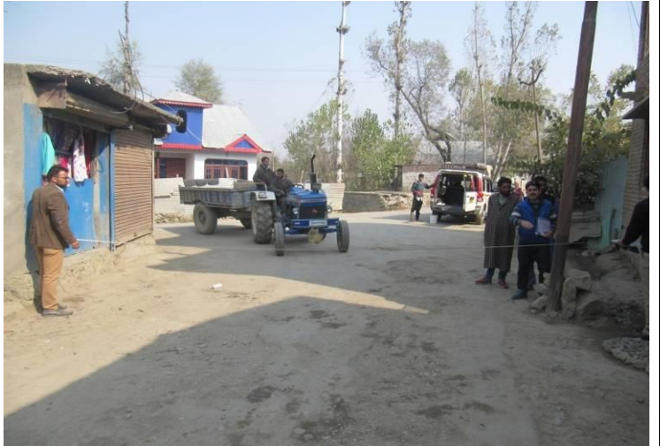
HARITAR JUNCTION PROJECT END POINT
